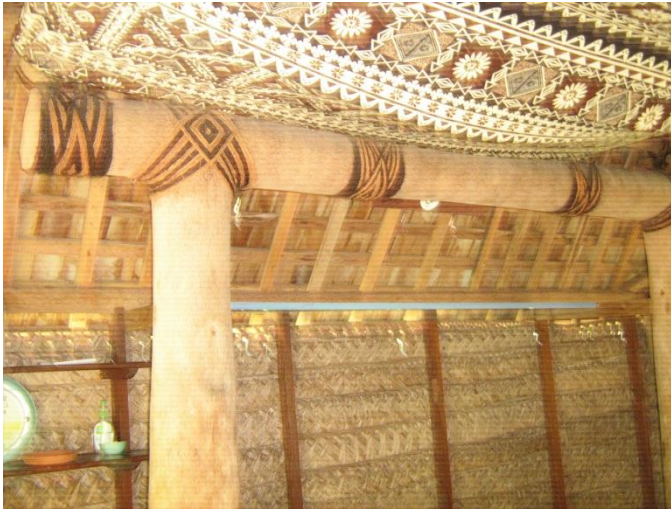
Ceiling and walls of a Fale
